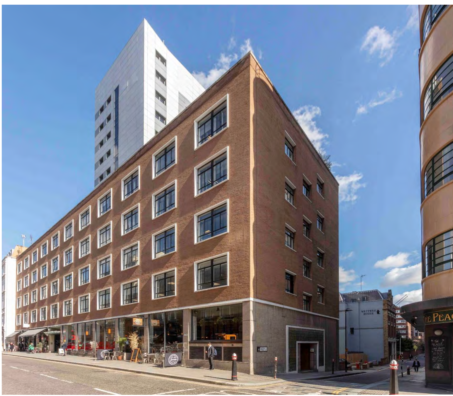
Photo: View from Minories towards northeast (Application site)
