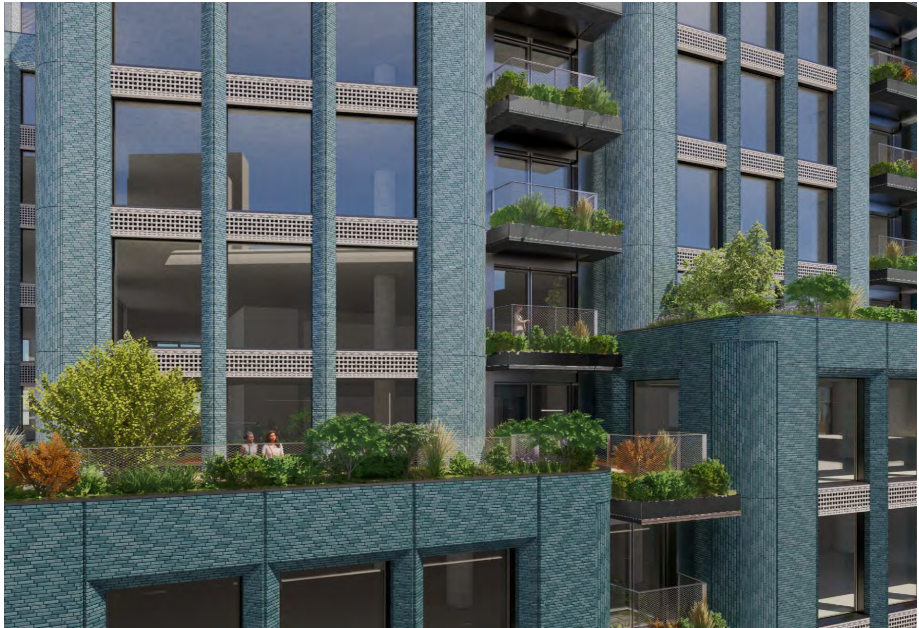
Bay details showing materials
